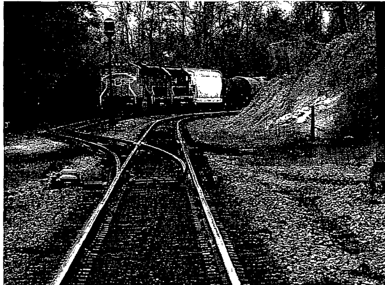
Figure 2: No. 15 turnout at siding
