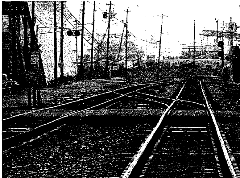
Figure 3: Intermediate Crossover near MP 667 (No. 10 turnout)
