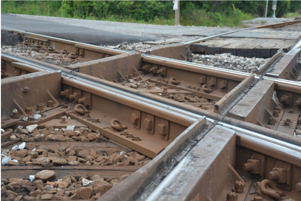
Canadian National crosses the CSX main line on a flange-bearing diamond at Mobile.
