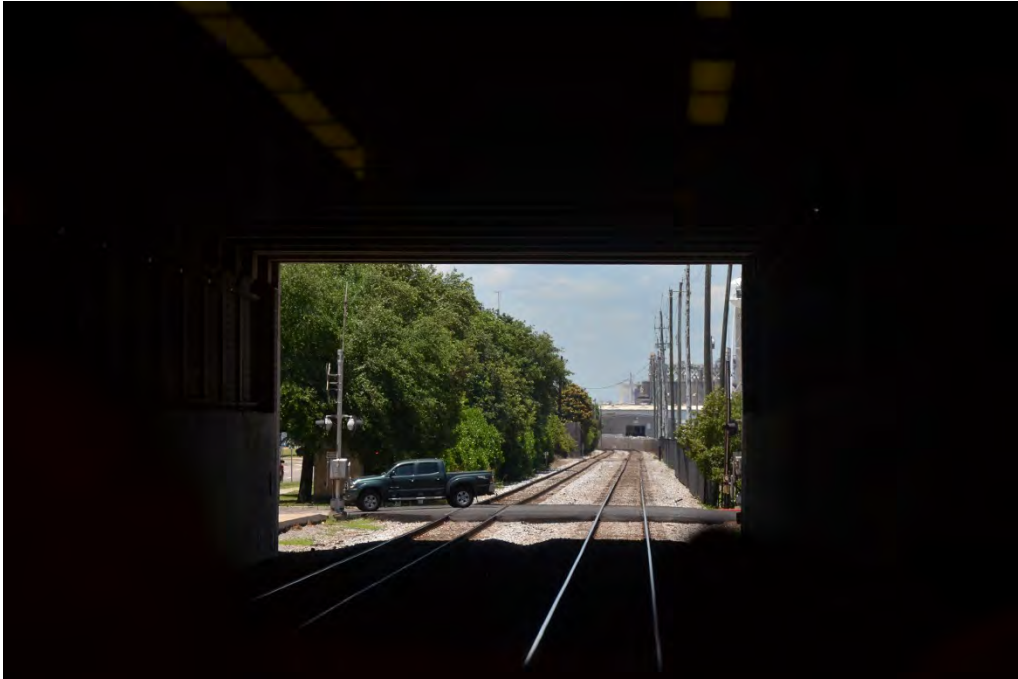
Framed through the Alabama Convention Center, the double main track NO&M Subdivision heads north toward Sibert Yard.
